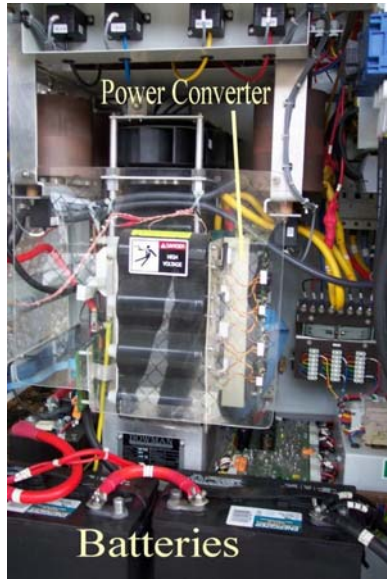
Fig. 3.4. Bowman inverter location.
