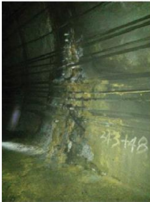
TYPICAL CABLES WITH VERY HEAVY CALCIFICATION
