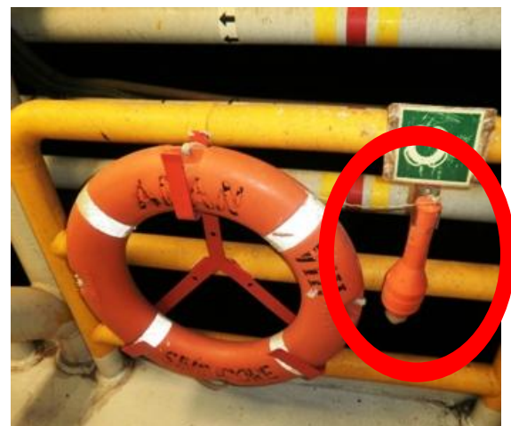
51- The rig has at present very poor quality of life saving equipment like ropes and flotation lights for ring buoy. These have to be replaced with standard equipment provided in the safety catalogue. Information for both these items is available in the Safety Catalogue Pg 100 & 101.
