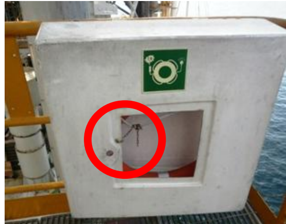
52- Bracket for the smoke buoy on port side is damaged and the pin to hold the ring buoy in the box is missing. A substitute pin should be installed to avoid losing the buoy.
