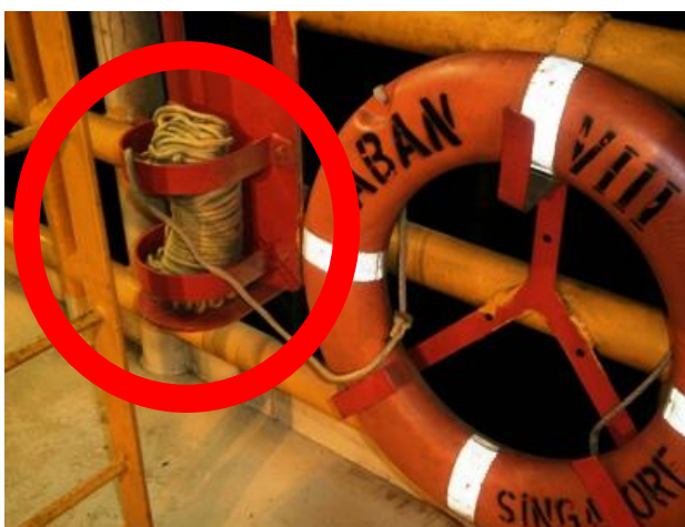
51- The rig has at present very poor quality of life saving equipment like ropes and flotation lights for ring buoy. These have to be replaced with standard equipment provided in the safety catalogue. Information for both these items is available in the Safety Catalogue Pg 100 & 101.
