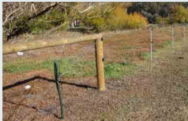
Figure 7.13 – Independent, short sections of fence where flows are expected to be particularly fast, and a point of potential avulsion
