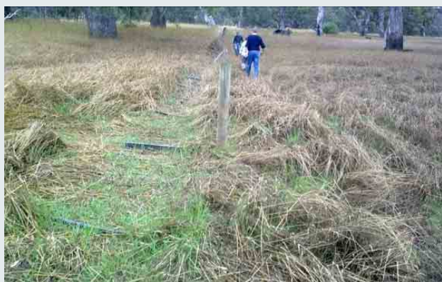
Figure 7.9 – Strained fence length in drop-down position (photo: Glenelg Hopkins CMA)
