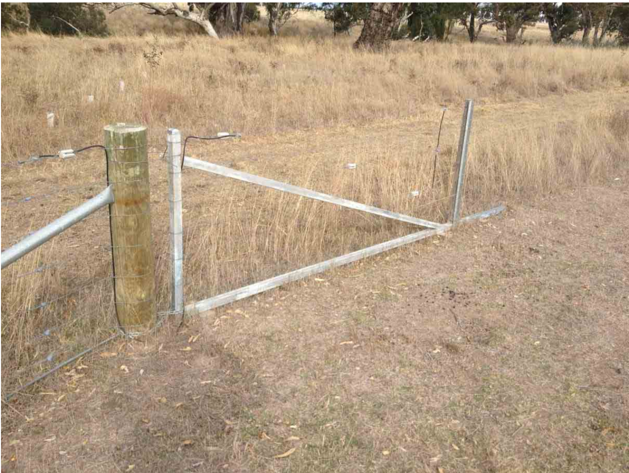
Figure 7.4 – Drop-down end assembly using chain in a figure-eight configuration as the bottom hinge
