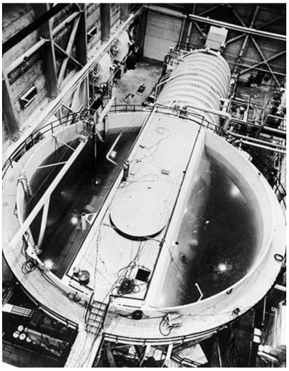
Reactor core for USS Nautilus undergoing tank tests (Credit: Idaho National Laboratory)
