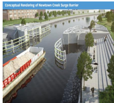
Conceptual Rendering of Newtown Creek Surge Barrier PlaNYC Brooklyn-Queens Waterfront, Chapter 14, p. 256 http://www.nyc.gov/html/sirr/downloads/pdf/final_report/Ch14_Brooklyn_Queens_FINAL_singles.pdf , MMR:
