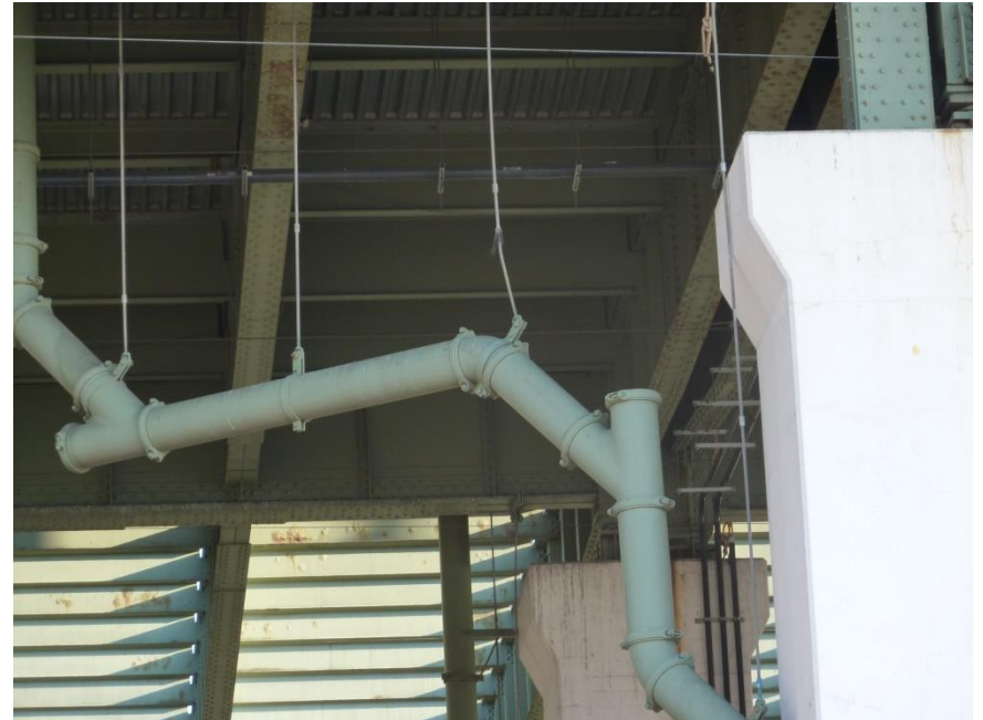
Drainage Line and Roadway Overpass
