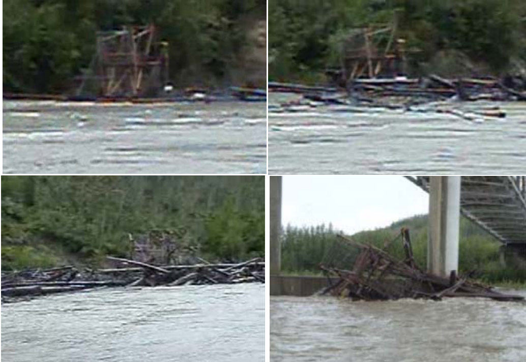
Figure 3: Large entangled debris event impacting (upper left) and carrying off (upper right and lower left) a fish wheel on the Tanana River near Nenana, Alaska, and depositing it against a bridge pier (lower right) (courtesy of Stephen Lord)
