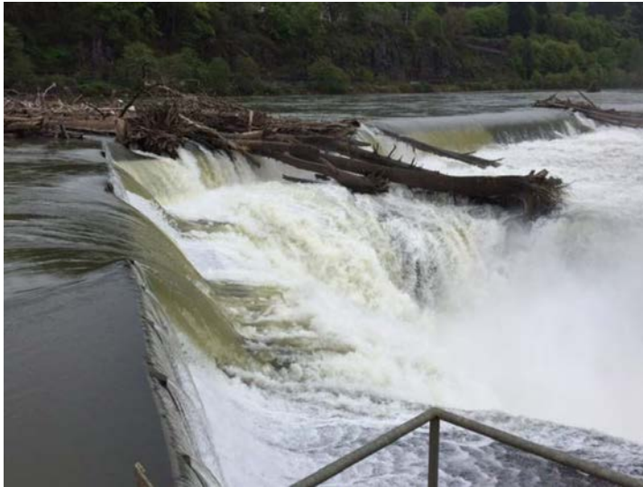
Figure 3. Photo of dam crest on 05/01/2017 showing flashboards in place and debris accumulation.
