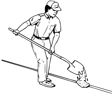
Figure 4.3 Placing Dirt on a Lateral
