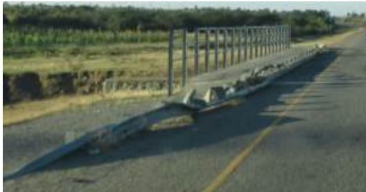
FIGURE 8 Badly damaged guardrail.
