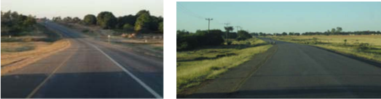
FIGURE 16 50-km/h zones along open highway with no abutting development or intersections.
