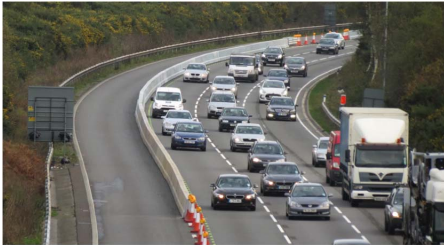
FIGURE 2 Temporary steel barriers.
