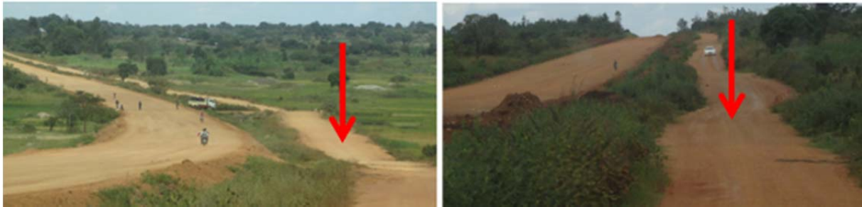
FIGURE 17 Temporary side tracks for the public while highway was being constructed.
