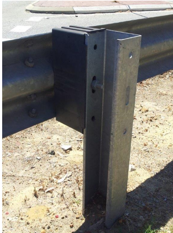
FIGURE 9 W-beam with solid plastic block out as used by Western Australia (viewed from behind the barrier).
