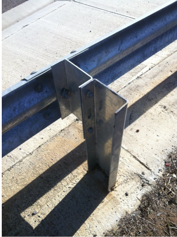
FIGURE 8 Type B W-beam system as used by Victoria and Tasmania.
