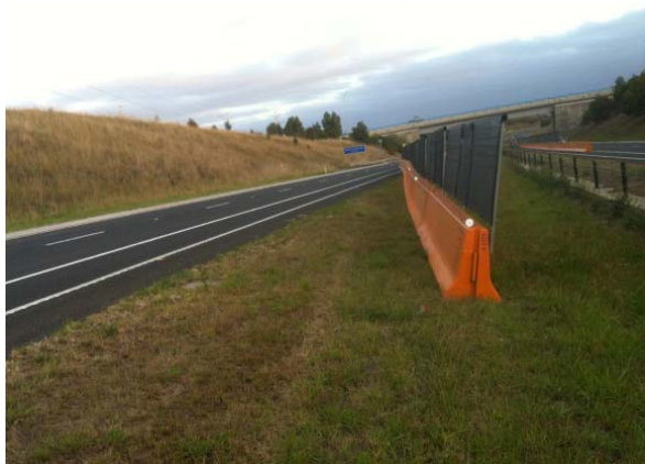
FIGURE 6 Barriers without an effective terminal ending in the clear zone.
