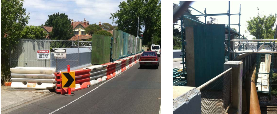
FIGURE 7 Plastic barrier protecting workers on bridge over a railroad.
