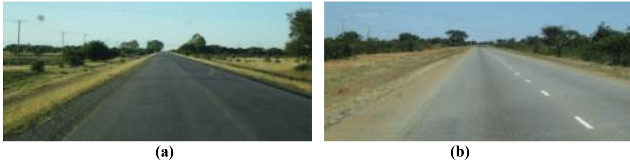
FIGURE 2 Typical cross sections: (a) no line marking and 1.0-m shoulder and (b) lane line marking and 1.5-m shoulder.
