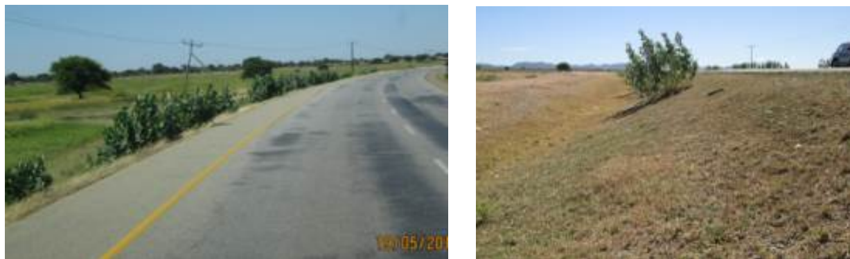
FIGURE 4 1:2 batter; 2 to 3 m high on a curve.
