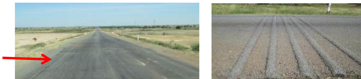
FIGURE 3 Nonvisible speed hump on open highway section with advance warning rumble strips.
