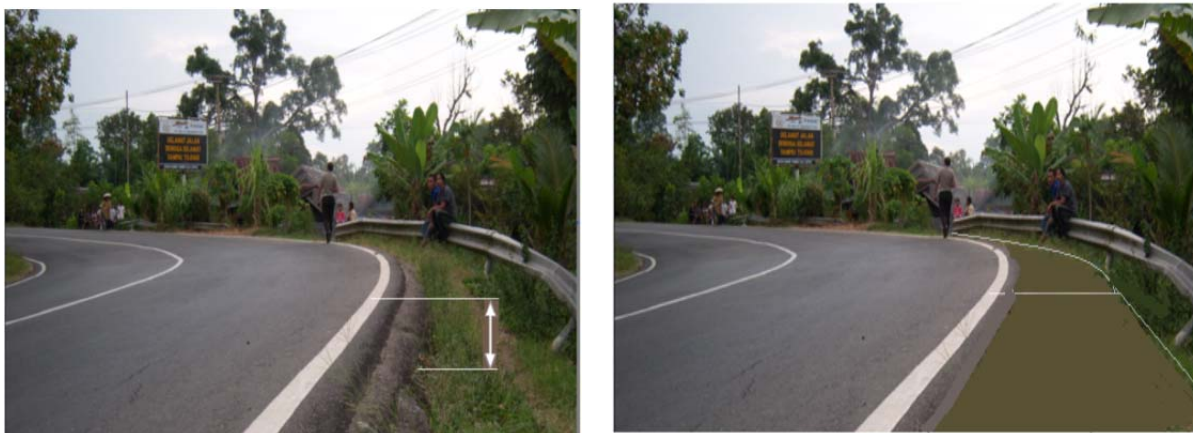
FIGURE 12 High gap of road edge and solution to improve road safety.
