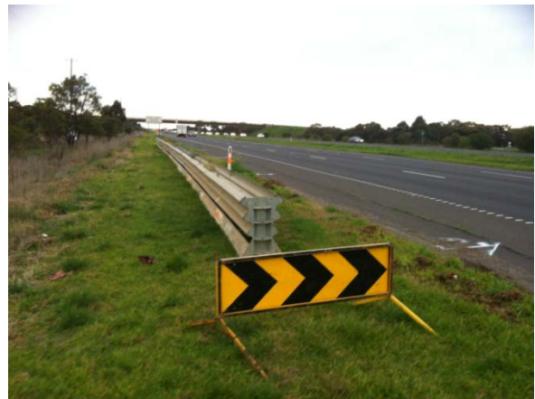
FIGURE 6 Barriers without an effective terminal ending in the clear zone.
