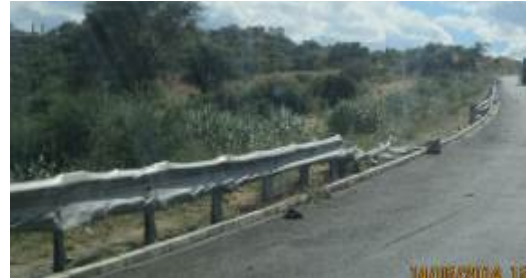
FIGURE 8 Badly damaged guardrail.
