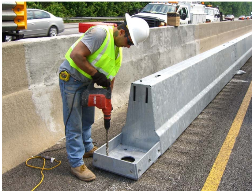
FIGURE 3 Pinning a barrier to reduce deflection.
