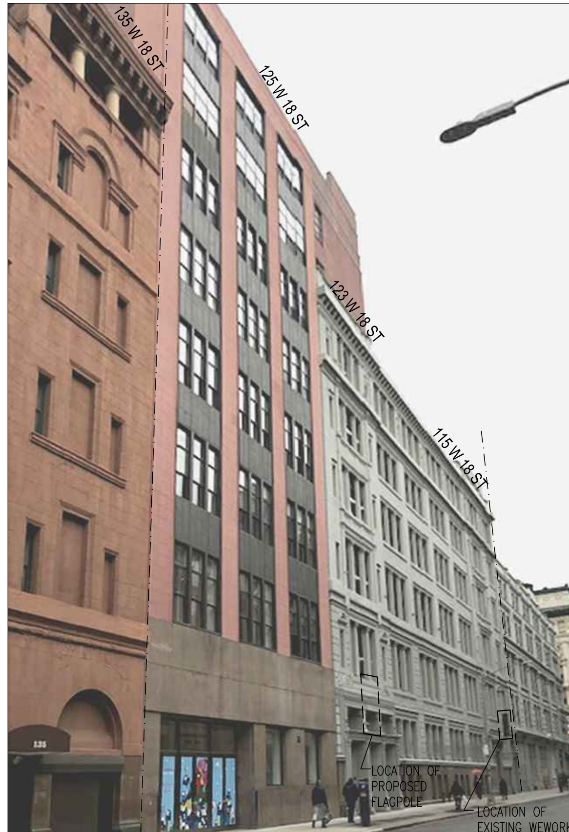
2 EXISTING CONDITION PHOTOGRAPH SCALE: NTS
