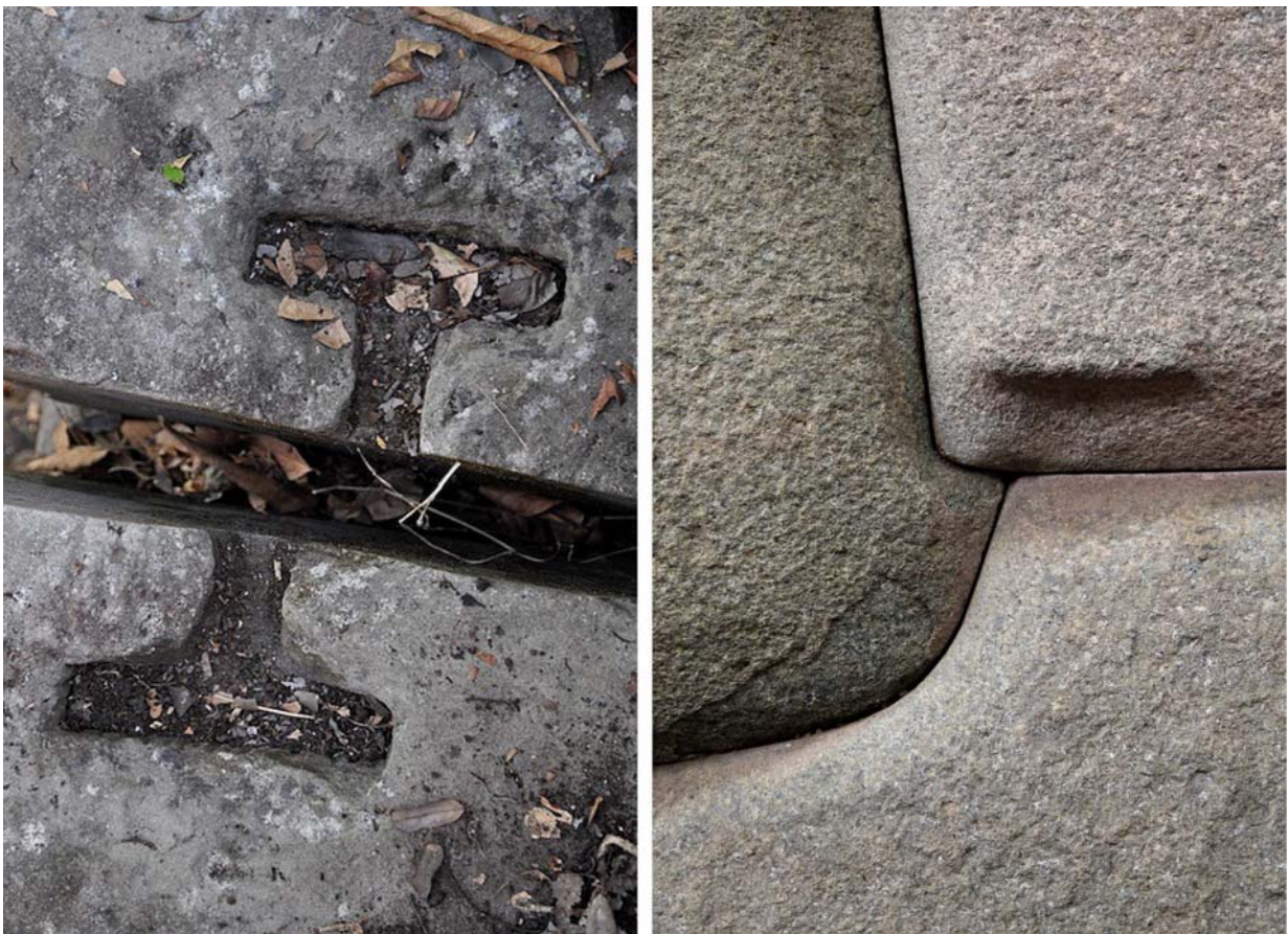
Figure 1. (a) Cavities that were carved into stones and fit with steel joints during the Angkorian era (Mitch Hendrickson, Source: Cambodia Daily), and (b) Inca wall assembly detail (Brandon Clifford).
