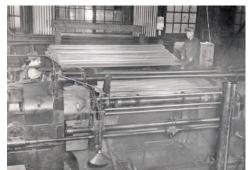
Threading pipe on both ends
