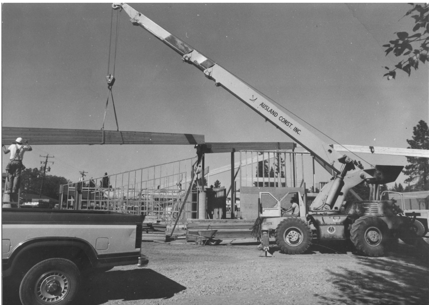
Coates Hall construction, 1980s
