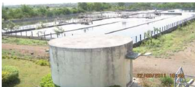
STP at Chehed, Nashik
