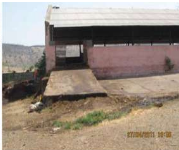
Abattoir releasing effluents and solid wastes
