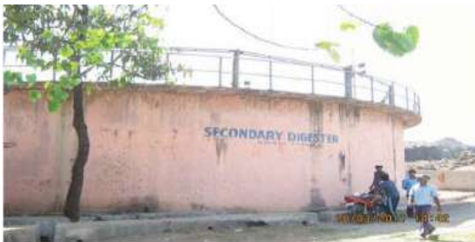
Secondary Digester of the STP at Adharwadi
