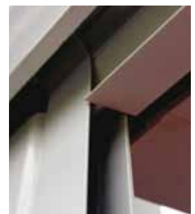
Guide & bottom rail interface
