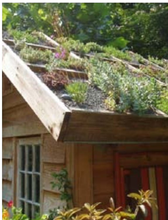
Example of a green roof. Amelio Ancaya, Living Roofs, Inc.
