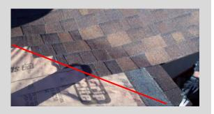
Lay a row of shingles so that the bottom edge just touches this line, as we had previously been doing on top of the valley flashing, and the edge of the starter strip.
