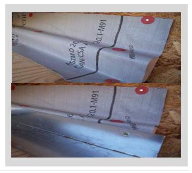
Attach the L flashing to the flashing nailer with 1- 1/4" roofing nails along the top edge of the metal. Always try to keep the nails as far from the bend in the L flashing as possible (Nail high). Do not nail into roof.
