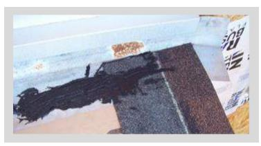
We are no longer using metal valley flashing on our roofs. The new procedure is done with shingles only and is detailed in the section on shingling. At this point all that needs to be done is to run a piece of underlayment down the valley.
