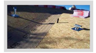
All roof penetrations require a galvanized metal roof jack. At this point verify once again that the proper jacks are on hand. These will be installed over the underlayment, and in between the layers of shingles. Install a second piece of underlayment (about 2 feet wide) over the top half of the jack flashing and extend it up under the next highest joint for further leak protection. Do not install the jacks until shingle installation.
