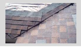
If your row of shingles ends at an L/Z flashing, the last shingle should end about 1/2" from the vertical leg of the L and no nails are to be driven through the horizontal leg of the L. Before installing the shingle lay a 4" wide bed of tar starting about 1" from the vertical leg of the L flashing and continuing out onto the underlayment. Now lay the last shingle, but nail only up to the edge of the L flashing. The tar bed will secure the remaining length of shingle.
