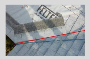
Now shingle and complete the higher roof as you normally would, starting each row at the inner edge of the valley shingle (as we had when using the metal valley flashing).
