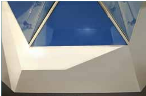
Interior view of a Lantern Rooflight 1200mm x 1500mm.
