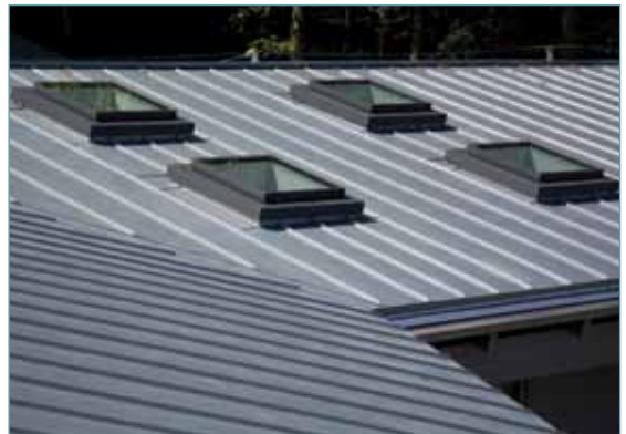
Castle Drogo, Devon. The Harrison Sutton Partnership specified a series of 900mm x 900mm Rooflights.
