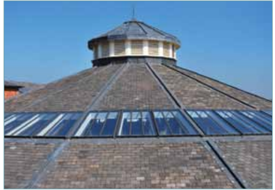
The Roundhouse, Derby. Maber Architects specified Bespoke Rooflight, Type A-Linked.
