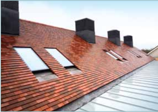
Broadclyst School, Devon. NPS South West specified neo™ Rooflights.
