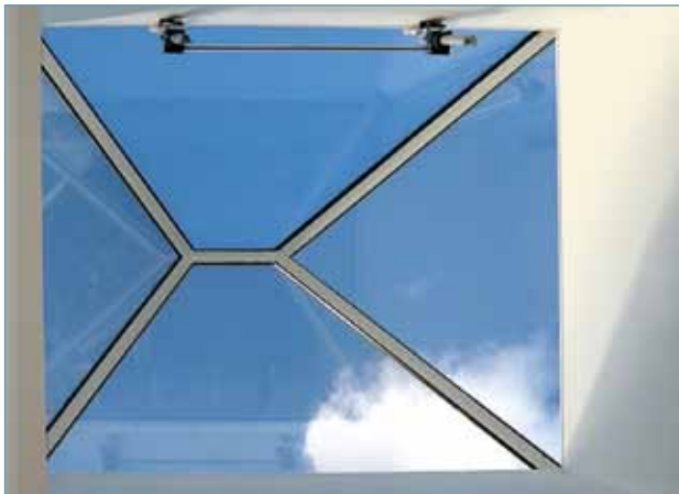
The silicone and Thermoliner® are white to blend with the pale interior on this Lantern Rooflight.
