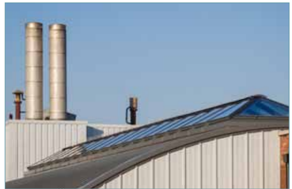
Robinsons Brewery Visitors Centre. A total of eighteen modular sections were joined together to create one large Lantern Rooflight.
