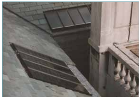
Somerset House, London. TGB Consult specified forty Bespoke Conservation Rooflights®.
