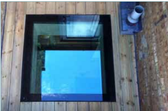
Residential Property Oxford. Walk on Rooflights allow natural light ingress to spaces below whilst creating a usable space above.
