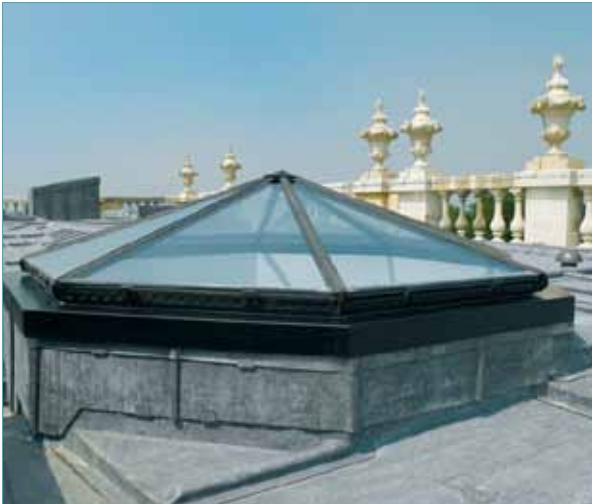
Ventilation is easily achieved by means of an electric actuator.
