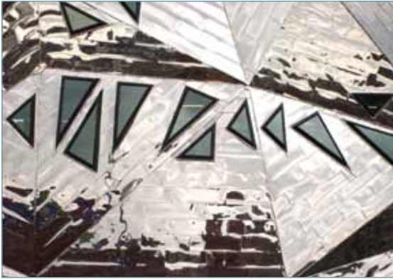
The Public, West Bromwich. Will Alsop Architects specified Bespoke Triangular Rooflights.
