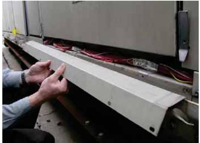
Figure 53: RFS and RCS Interconnecting Control Wiring
