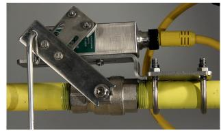
Figure 18. Safety Shower Valve in Activated Position
