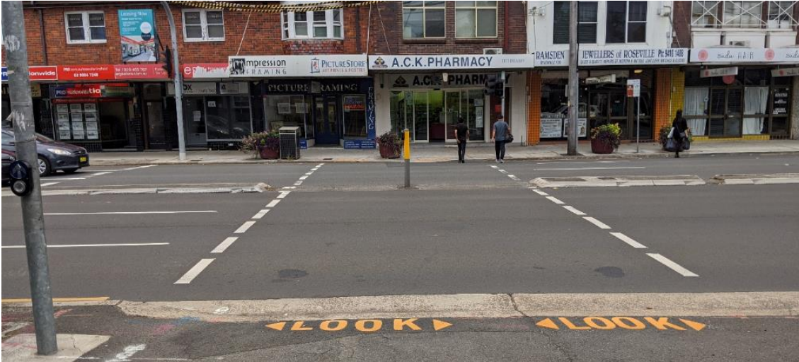
Figure 2.15 Pacific Highway signalised crossing (P4)
