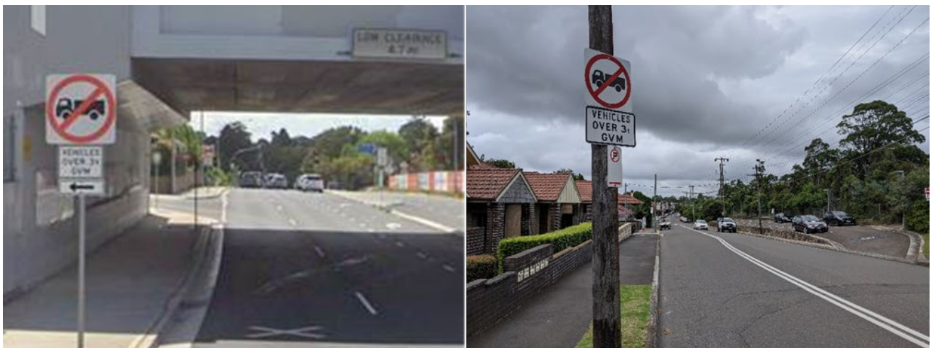
Figure 4.1 Hill Street weight limits and overbridge
