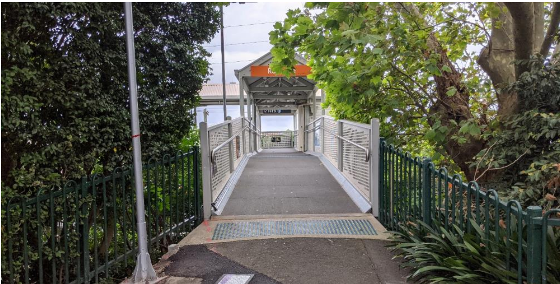
Figure 2.16 Graded access to overpass from Pacific Highway (P5)
