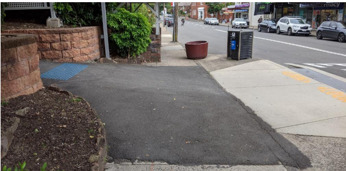
Figure 2.13 Graded access to station on Hill Street (P2)
