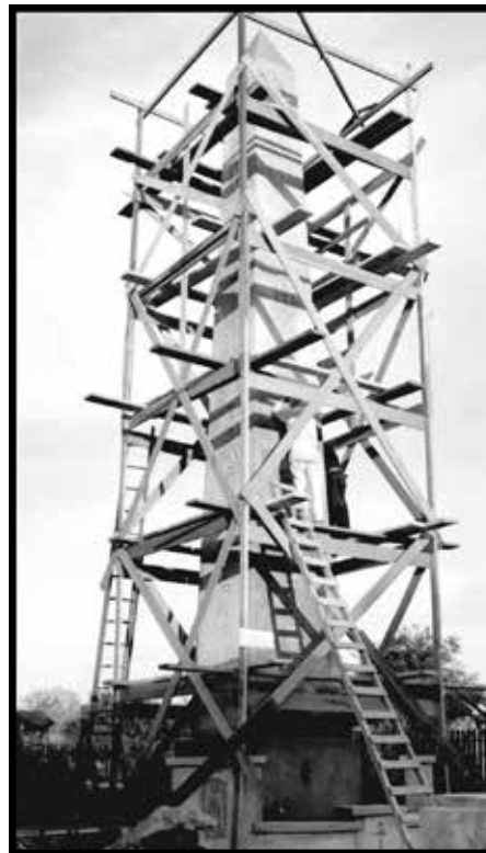
H. Spencer Lewis on "Reaching the Roof": "I allowed my mentally-created structure to tower into the skies to enormous heights..." symbolized by Rosicrucian Park's obelisk in the process of being placed into position, 1937.
