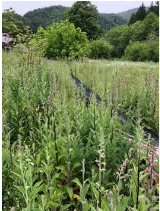
Figure 3-28 Sediment fence should be removed once vegetation is established
