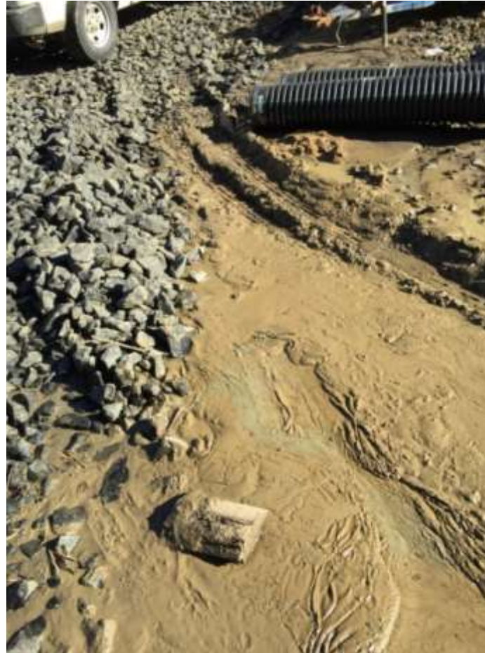
Figure 2-6 Sediment Non-Compliance
