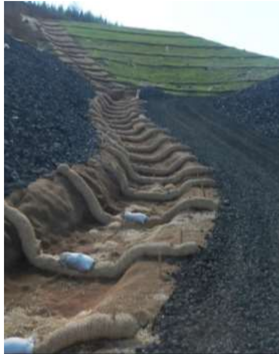
Figure 2-12 Stabilized Channel
