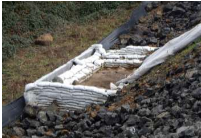
Figure 2-13 Sediment Trap & Energy Dissipater W/ Level Spreader
