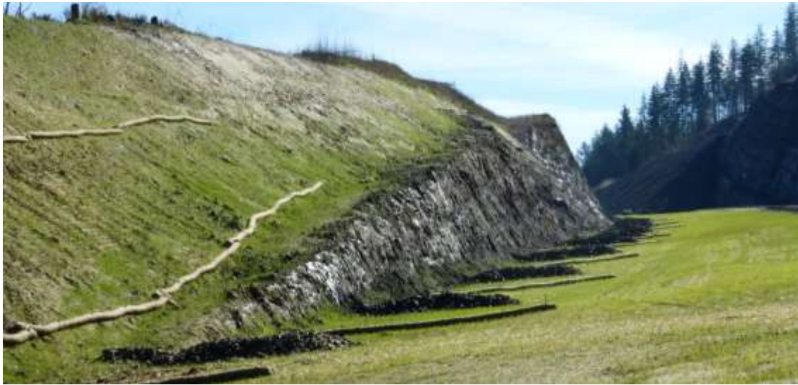
Figure 2-1 Good Sediment Control
