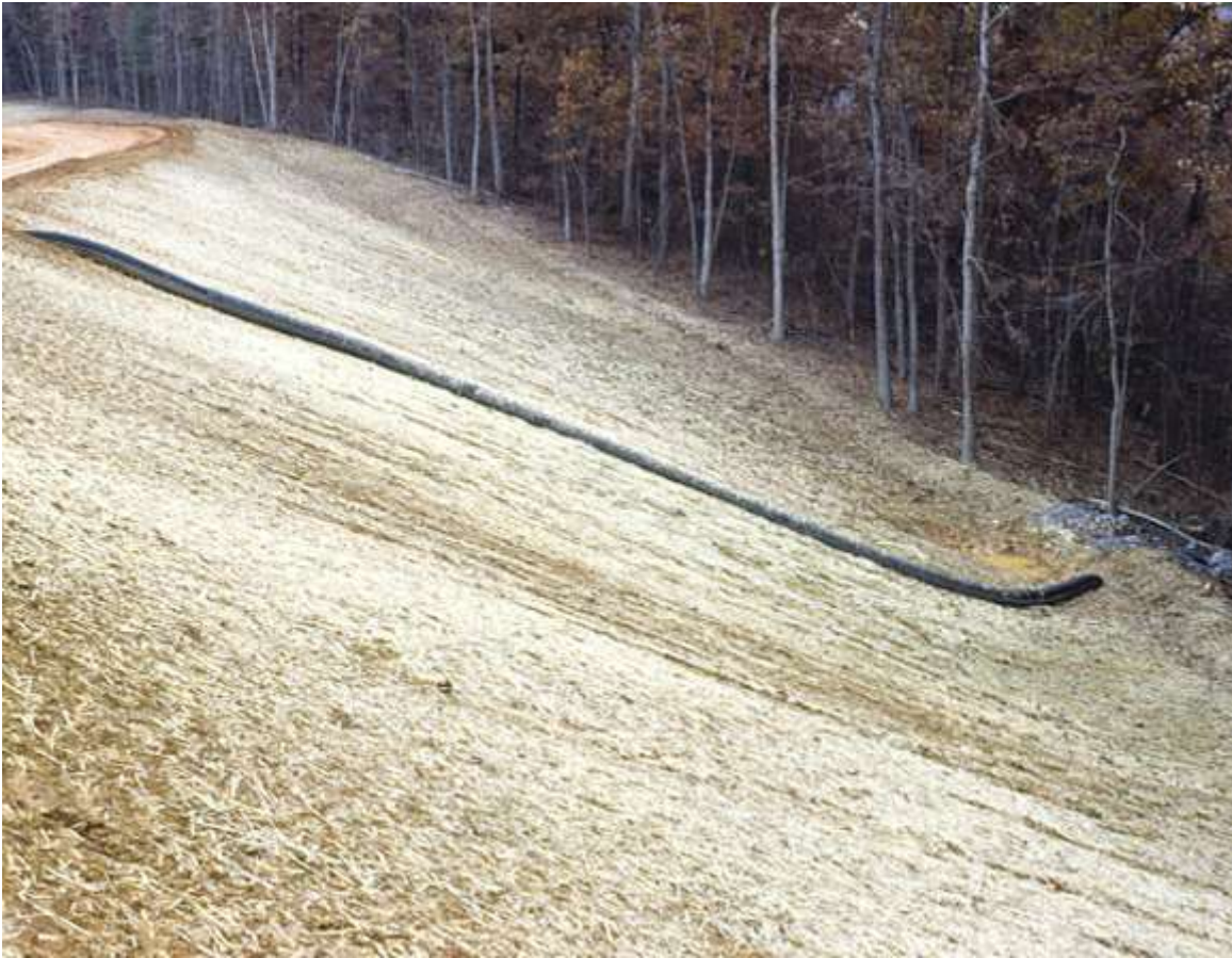
Figure 3-14 Temporary Slope Drains
