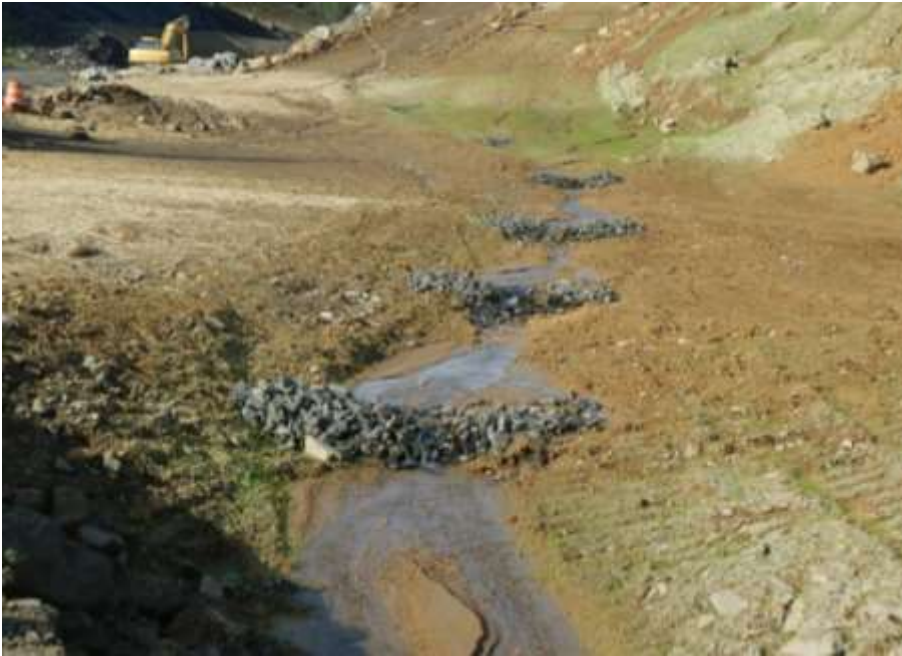
Figure 3-18 Check Dam
