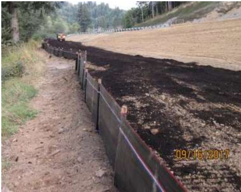
Figure 3-27 Sediment fence is trenched in correctly
