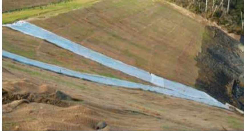
Figure 3-13 Plastic sheeting runoff control on slope matting
