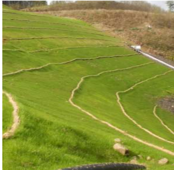
Figure 2-10 Seeded perennial rye grass with wattles to shorten slope length
