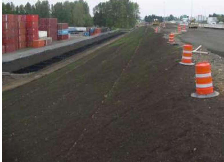
Figure 3-12 Compost blankets provides erosion prevention
