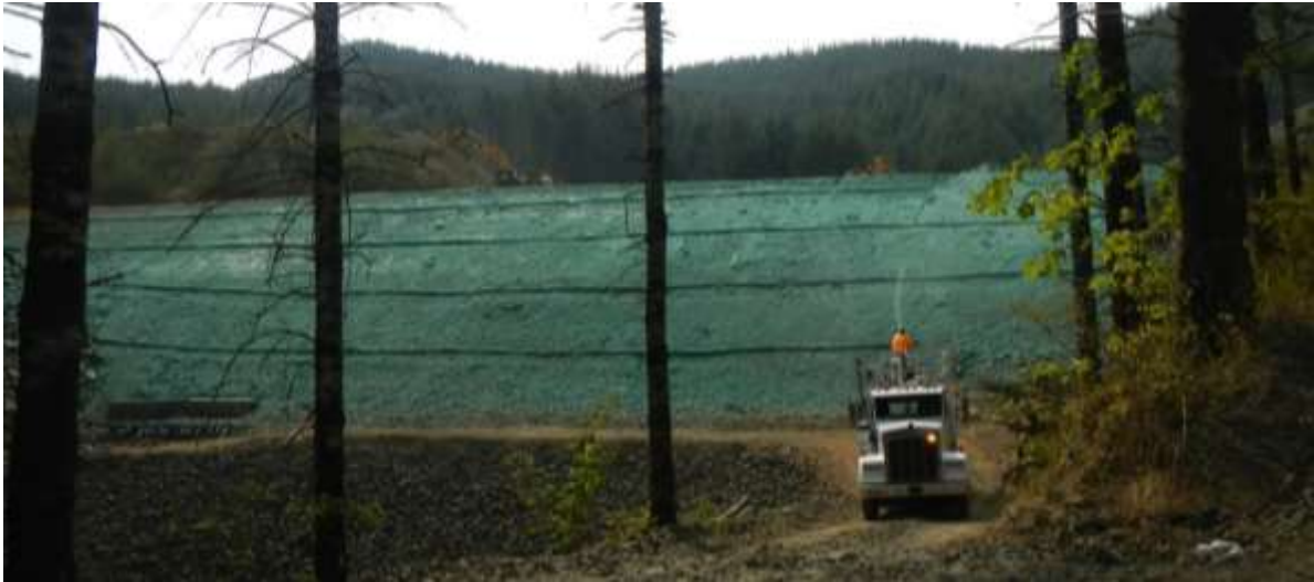
Figure 3-4 Seeding & mulch applied with Hydroseeder
