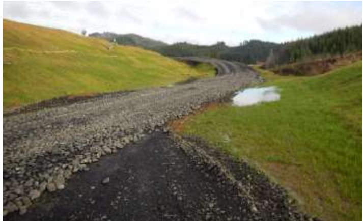
Figure 3-21 Stabilized Haul Road
