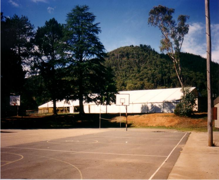
'Erecting the mess hall'
