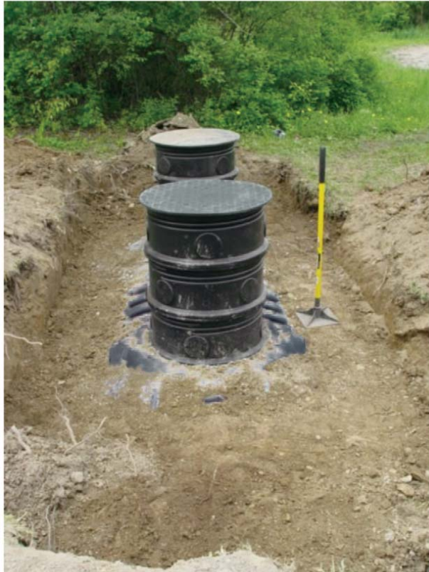
Photo 4.1.11-Example of evenly and uniform backfilling with native material
