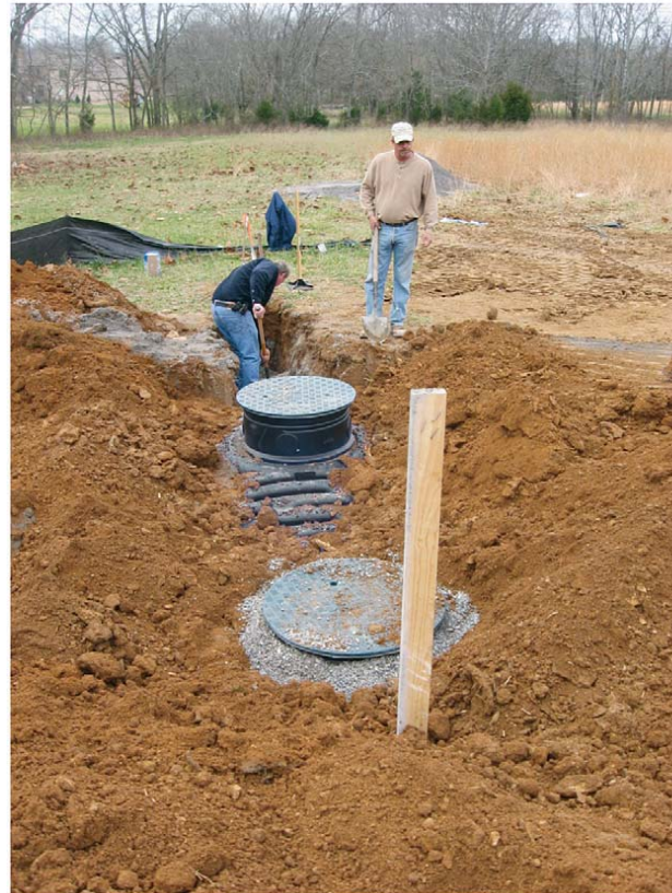
Photo 4.1.12-Example of complete backfill
