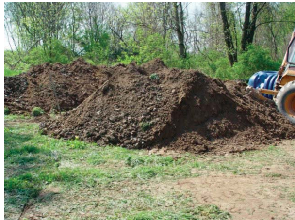
Photo 4.1.10-Example of backfilling material
