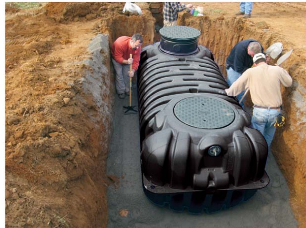
Photo 4.1.6-Spreading & compacting of backfill material
