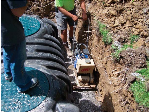
Photo 4.1.8-Example of mechanical compaction
