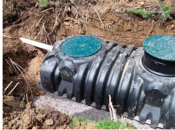
Photo 4.1.9-Uniform level distribution of material
