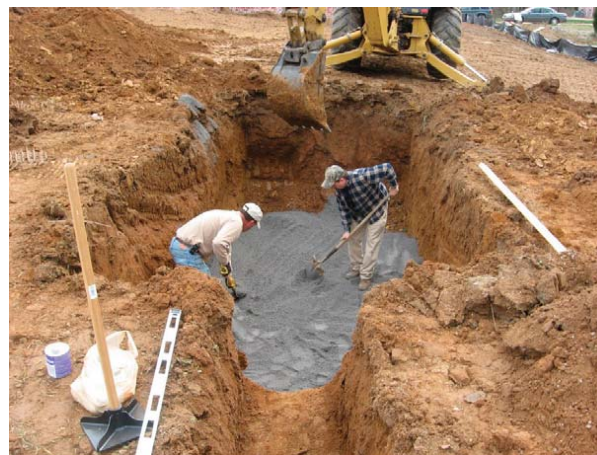
Photo 4.1.3-Bedding being spread and compacted
