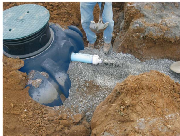
Photo 4.1.15-Example of careful and uniform backfill of piping system
