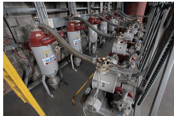
Photo 2.3.3– The new material handling assembly
