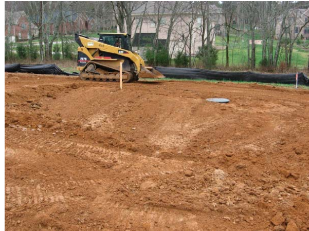
Photo 4.1.14-Example of final grading
