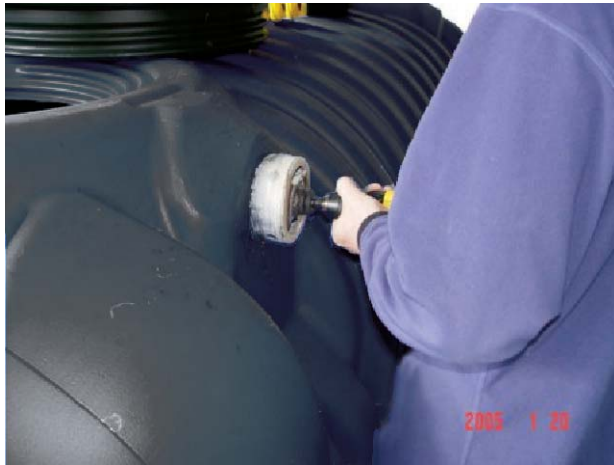
Photo 4.1.1-Drilling of inlet and outlet holes
