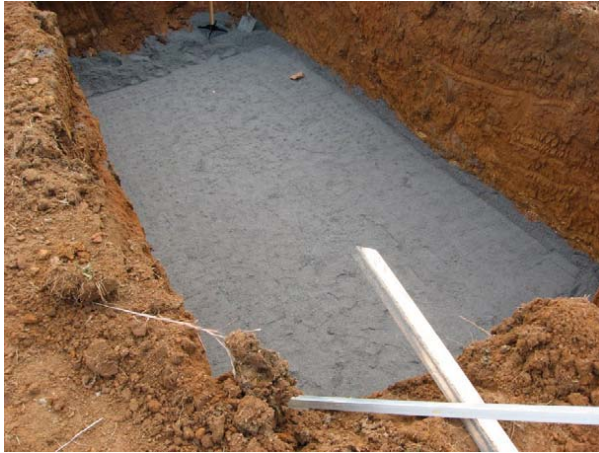
Photo 4.1.4-Bedding material prepared for setting the tank
