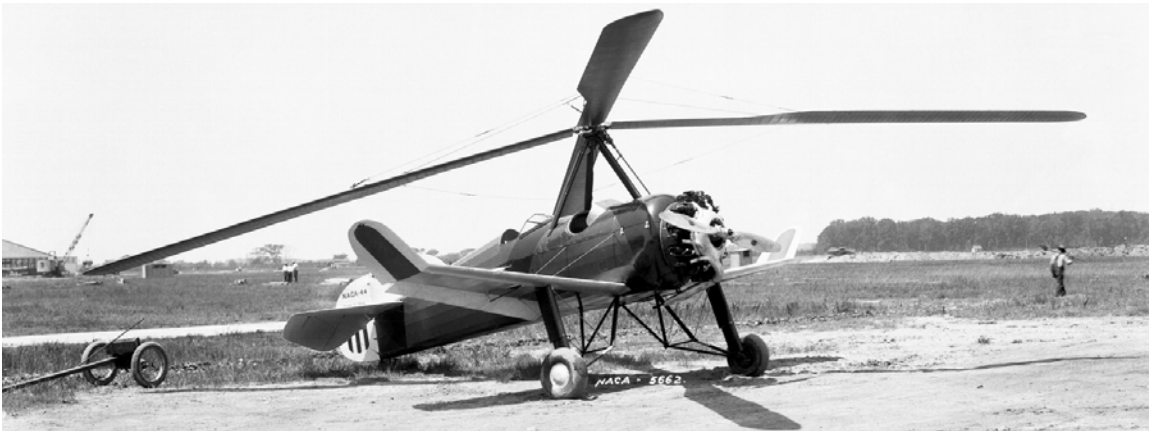
Fig. 2-1 The Pitcairn PCA-2 autogyro popular in the early 1930s. N.A.C.A. used this aircraft to pursue its slowed rotor technology. At high speed, the rotor advance ratio approached 0.7.
