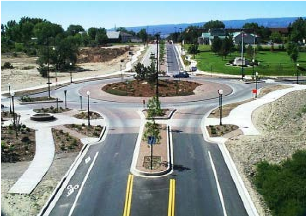
Figure 3.55– Example Pedestrian and Cyclist Treatment (Source: NCHRP 672 2 )
