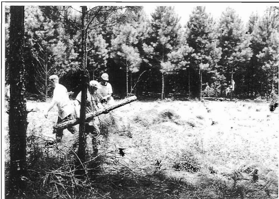
Figure 23. Clearing the planted pines in Area 8 for Blocks 1 and 2, view to the north.
