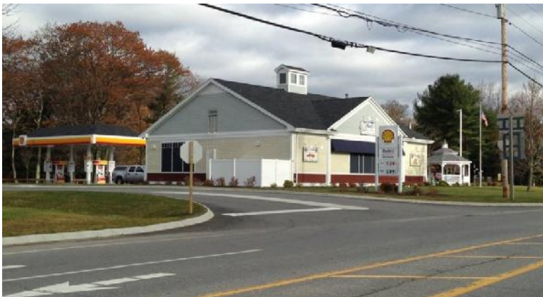
Gas canopy located behind the main building.
