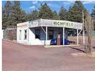
Front of Pine Breeze Inn, office, gas station and cabins, 1947 Route 66, Bellemont, AZ. The Pine Breeze Inn is at: N 35 13.452 x W 111 48.036'. February 24, 2006. NAU.PH.2004.11.2.423
