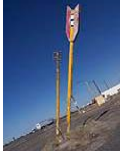
Deteriorating arrows, Twin Arrows Trading Post, 1947 alignment of Route 66. March 10, 2007. NAU.PH.2004.11.2.784
