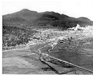
Williams, AZ. Intersection of the Santa Fe Railway mainline and the railroad to Grand Canyon. NAU.PH.94.34.4
