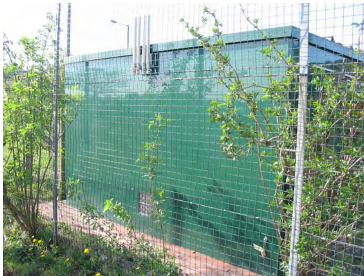
Figure 8.3 GRP kiosk. Grilles can be seen at low level
