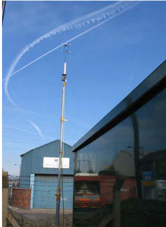
Figure 8.5 Ultrasonic anemometer positioned adjacent to the kiosk
