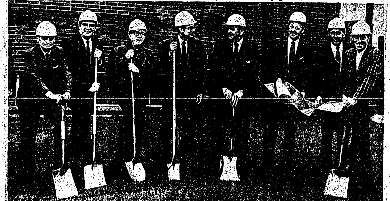
Building For Youth. Members of the Board of Commissioners of the Niles Park District get help last Sunday from members of the architectural firm and construction company as ground was broken for construction of an addition to the Niles Recreation Center administration building and for a recreation center at Oakton Manor park.
