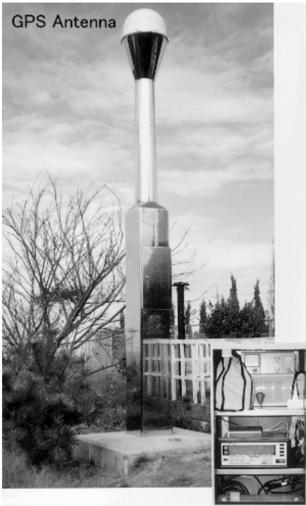
Photo 1 GPS-Based Control Station
