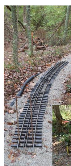
aid in keeping the radius in line and these were invaluable. The tie plates on both the short-approachtrestle and Bandy bridge had to be cut and rail repositioned for final welding. It was not easy but the radius was maintained.
