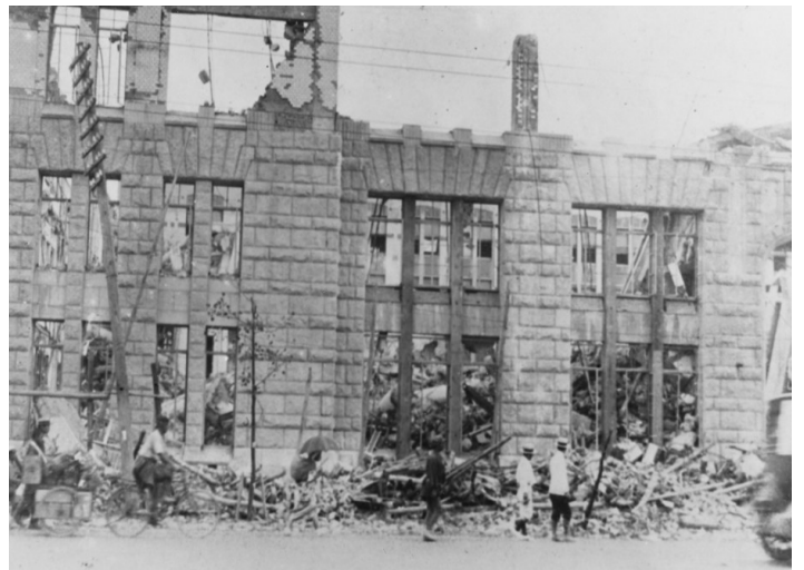
One wall standing and piles of rubble from what is left of the Yokohama Naval Hospital. (Naval History and Heritage Command, NH 91404)
