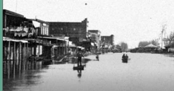
Regular flooding in Sacramento before the levee system was built (courtesy of CSH).
