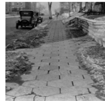
Concrete tiles, KCMO
