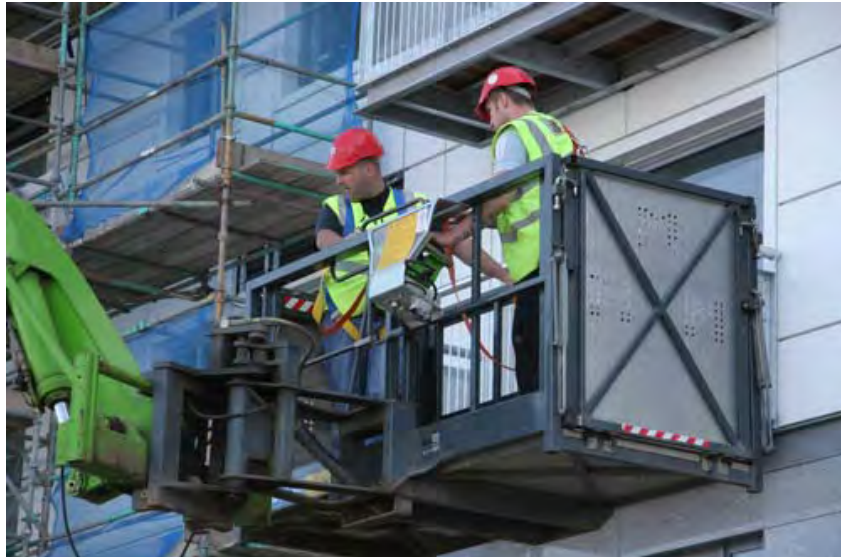
Figure 26 - Integrated Work Platform
