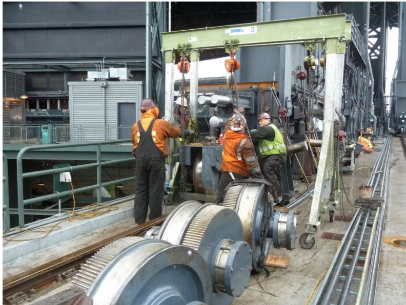
Interim Wheel Assembly Installation
