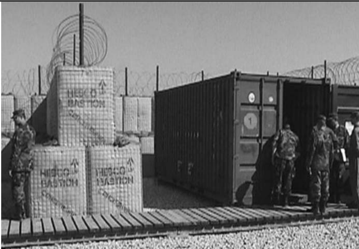
Figure 2-5. Example earth-filled barricade
