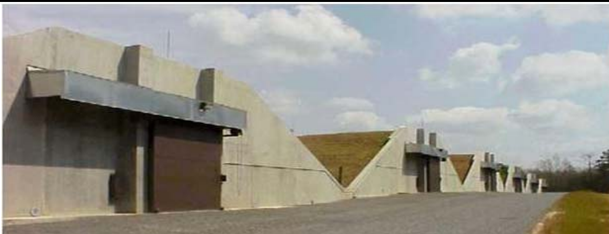
Figure 2-1. Example earth-covered magazines
