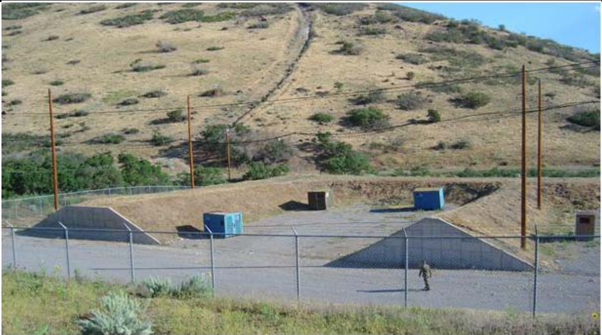
Figure 2-4. Example of revetted barricade storage pad
