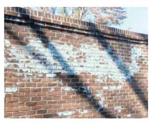
Figure10.2: Wall with Efflorescence
