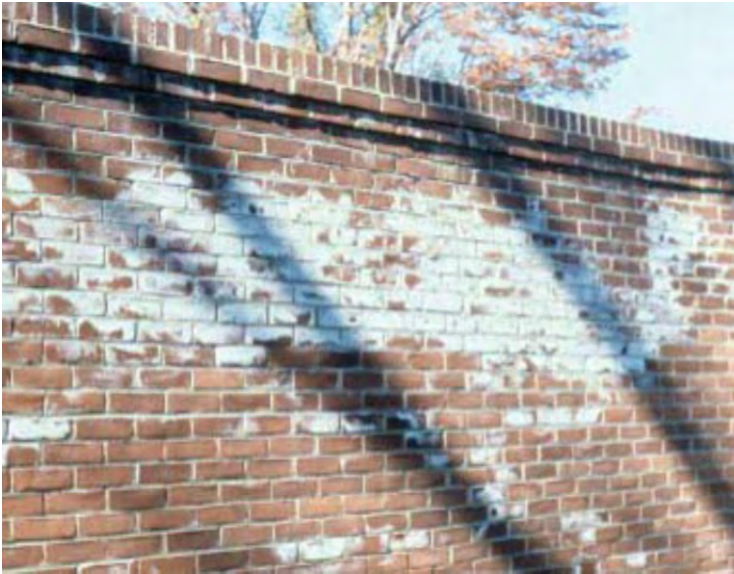
Figure 5.2: Wall with Efflorescence
