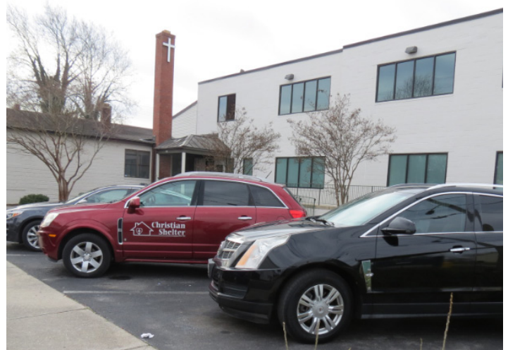
East wall renovations completed
