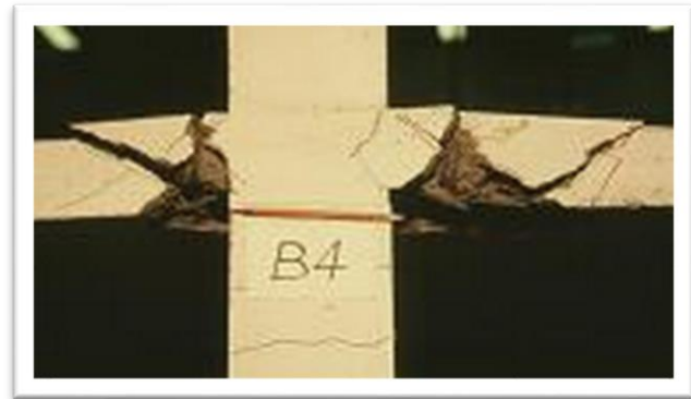
Figure 7. Yielding of slab reinforcement for a post tensioned concrete flat slab column.
