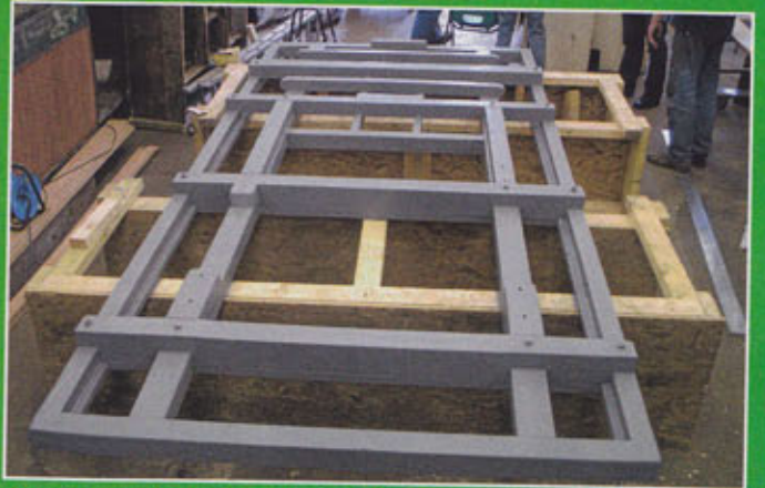
The new frame, utilising as much original timber as possible.
