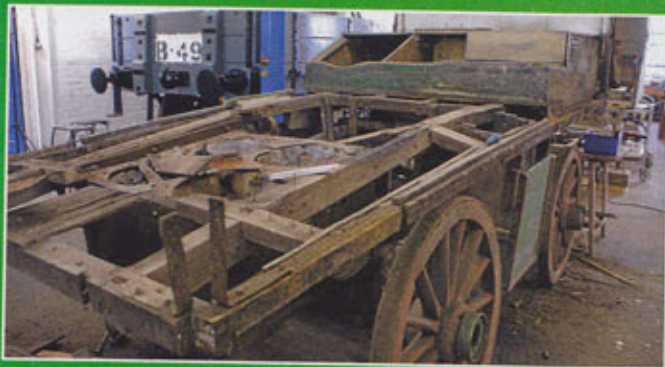
Upon strip down, the original frame is bared. Note the positions of the four coke-fired cooking wells.
