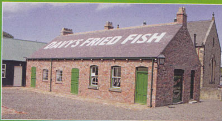
Beamish's new chip shop, made of brick to a traditional design. The typical provision in a pit village such as is recreated at Beamish would probably have been based in the front room of a terraced house. This format wouldn't be able to handle the demand so the next 'shop up' was chosen, and it can be imagined that a proprietor has occupied a former stables building and further expanded his business with an attached saloon in corrugated iron.
