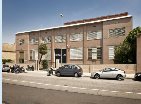
KITZ Corporation of Europe, S.A., Barcelona Plant, Spain
