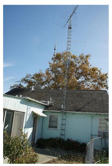
lowered. A few "easy does it's," my hand over hand release of the rope and what was fifty feet in the air is now lying on the ground. The Gin Pole is moved downward one mast section, the process is repeated until all the antennas are removed and only a naked tower still stands.
