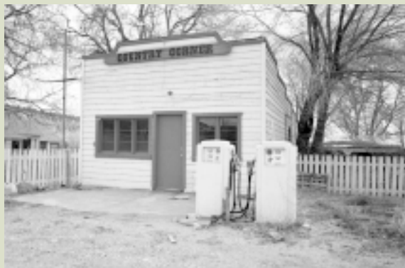
- Old gas station in Boulder, Utah, alongside Scenic Byway 12
