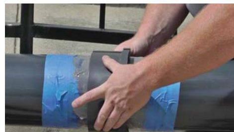
Position, Press & Hold Split Flange
